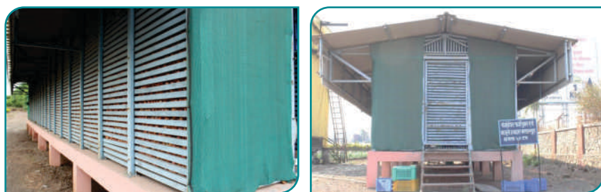
Fig. 9 Onion storage structures
