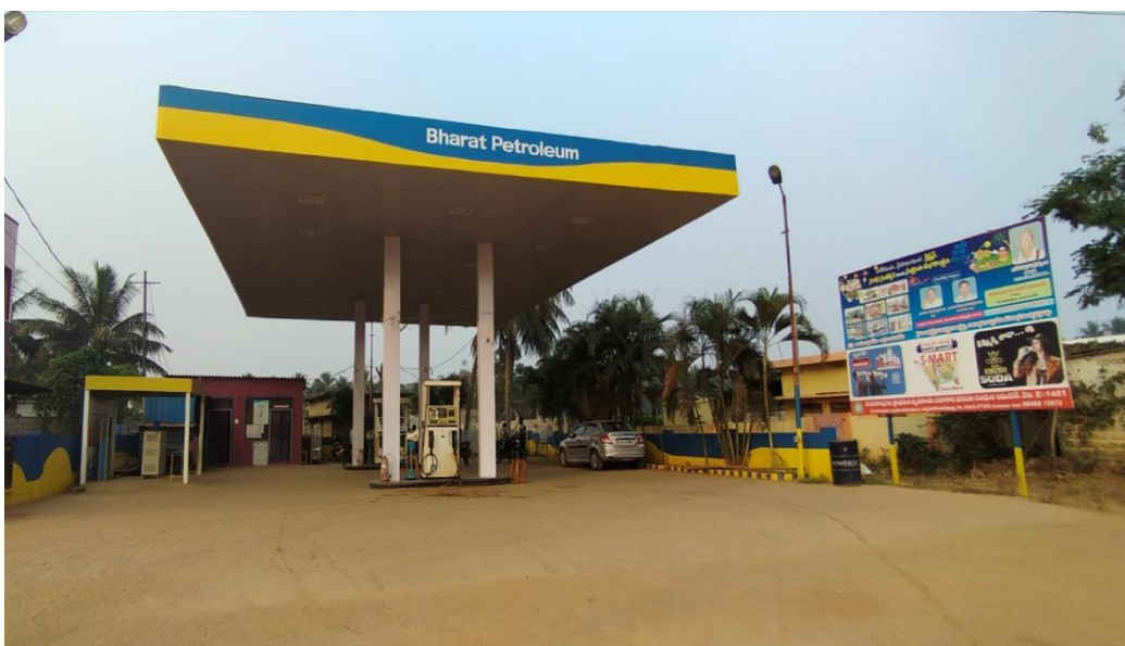
Fig. 10 Petrol and Diesel Pump
