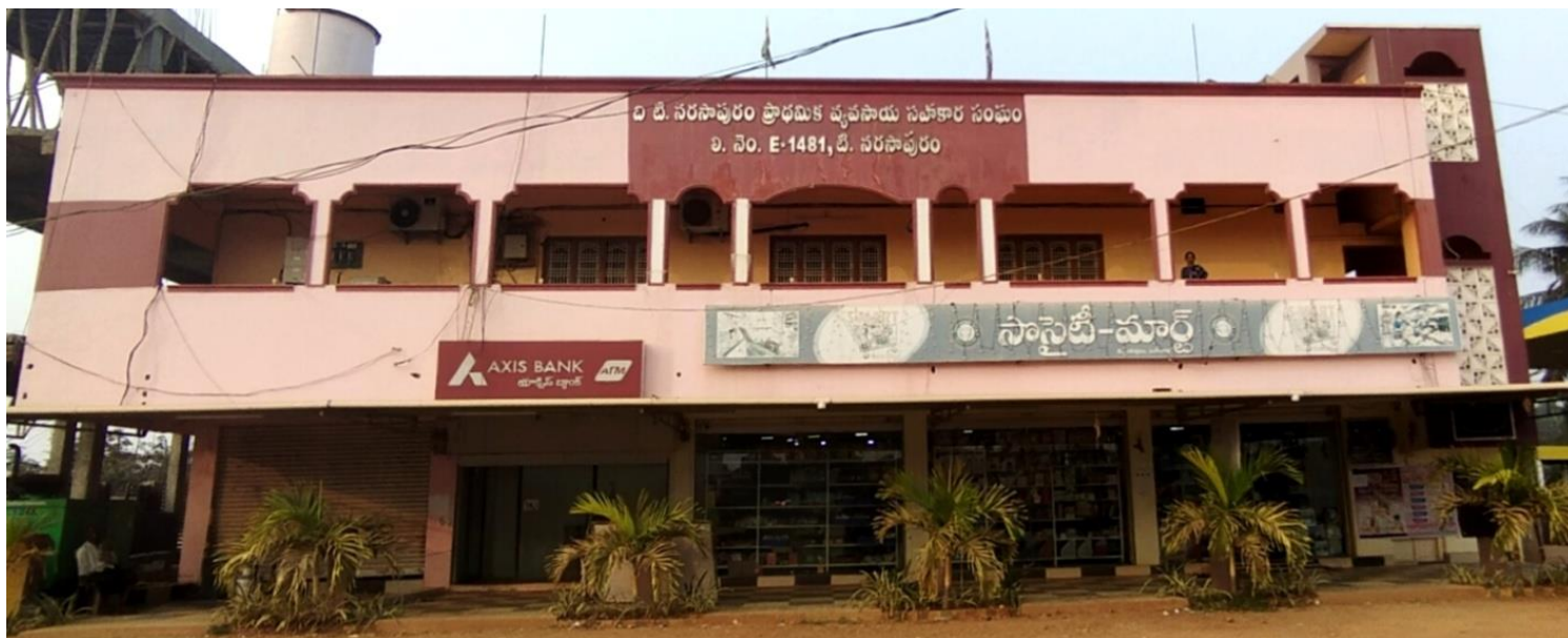
Fig. 2: T Narsapuram PACS Office Building
