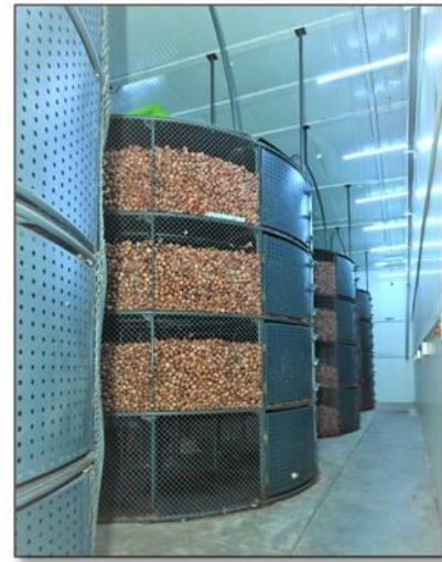
Fig. 8 Controlled Onion Storage Structure at Kala Biotech
