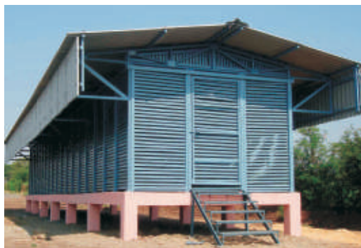
Figure 16: High volume bottom and side ventilated onion storage structure
