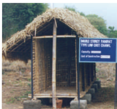
Figure 15: Low volume low cost onion storage structure
